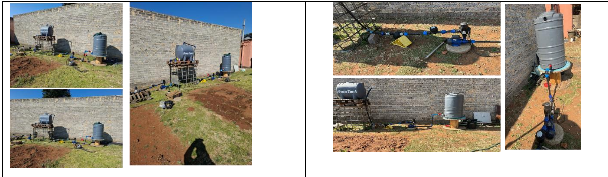
Figure 4: Various views of the wastewater treatment set up.
