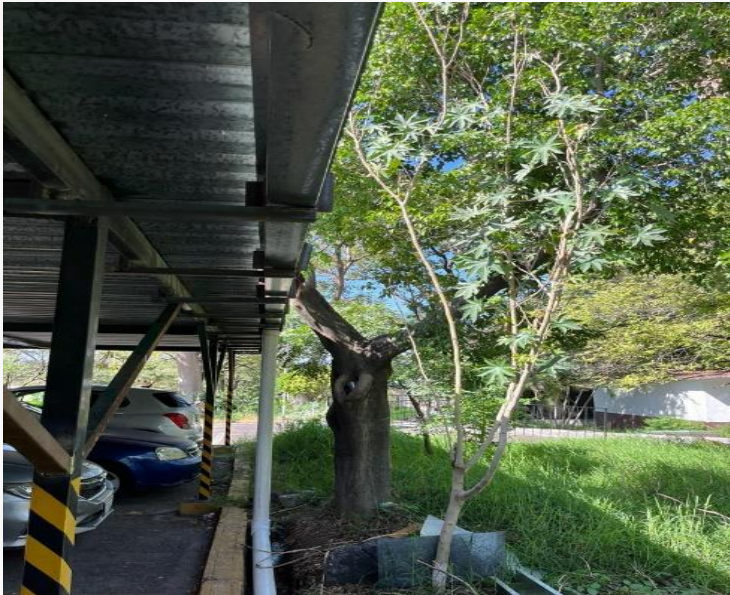
Gutters and Downspouts
