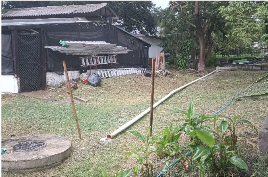
Discharge from the 6-inch SC1-2 pipeline
