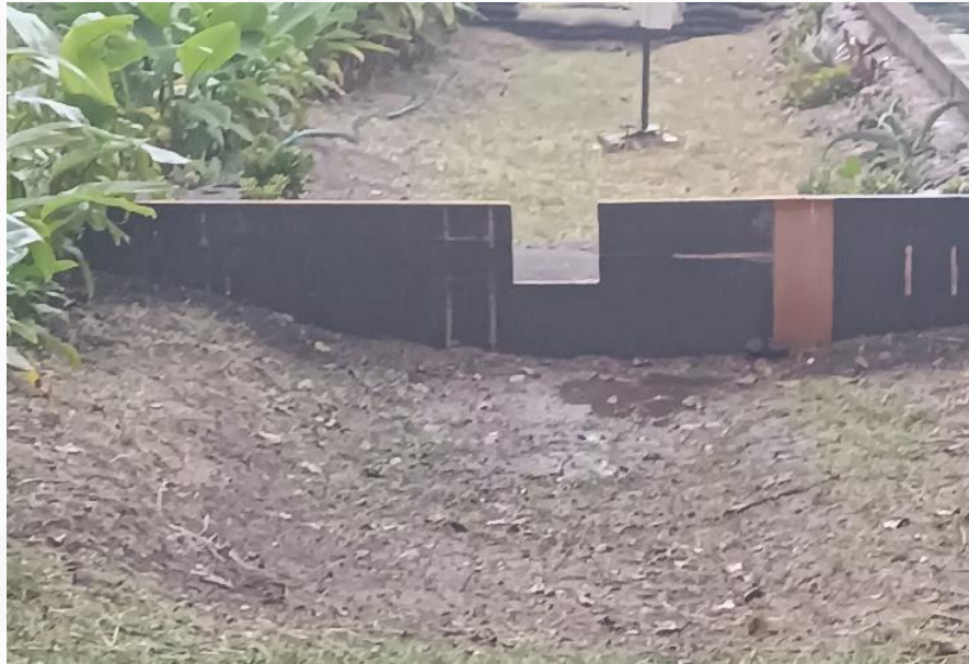
Spillway in SC2
